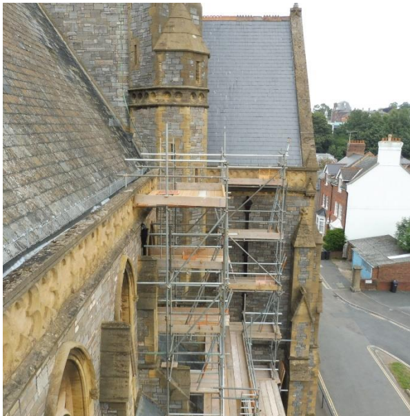
The scaffold erected along the south aisle
