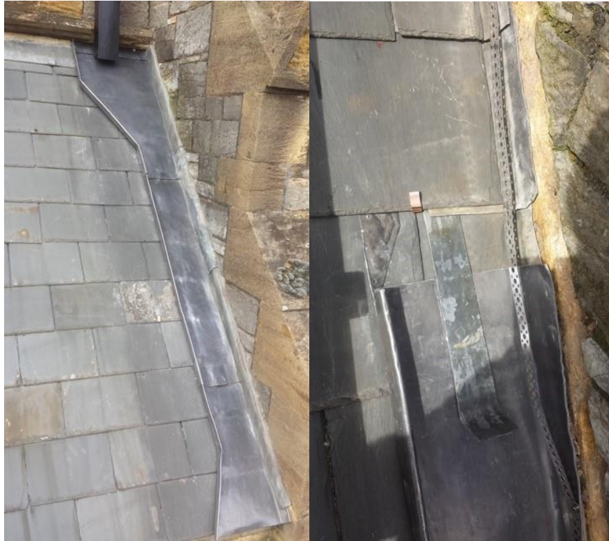
New lead 'chute' gutters over aisle roofs
