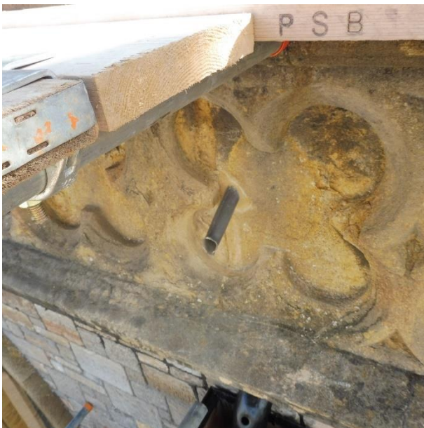
New lead drip detail from overflow gutter
